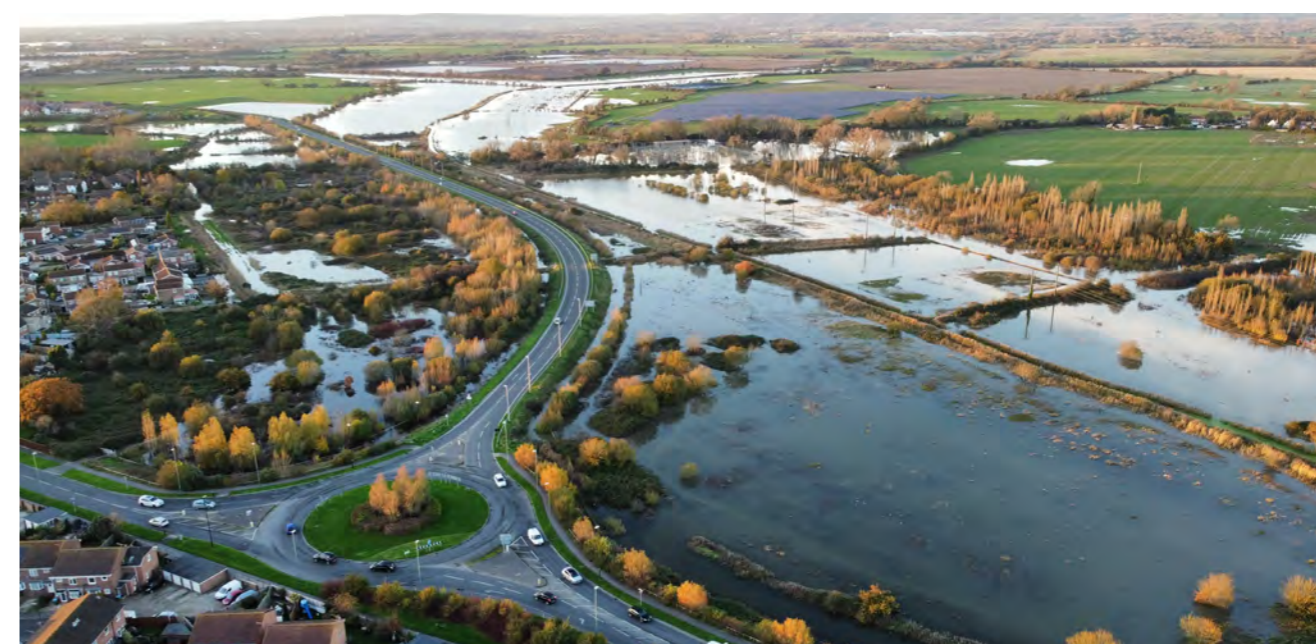
Key challenge - Flooding and future adaptability. Photo by Keir Greenway (17th Nov 2022)
